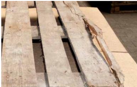
Diagonally, transversally or partially broken board
